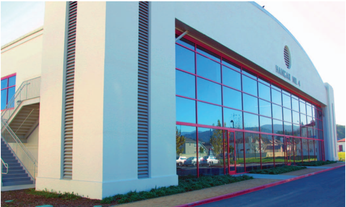
Exterior of Hamilton Landing project, which is a retrofit of a 70-year-old Air Force base hangar.
