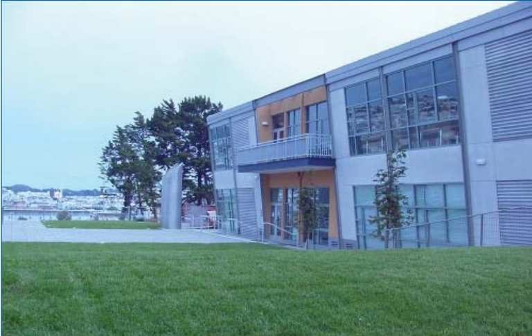
The exhaust pipe from the lower-level industrial arts classroom doubles as an exterior architectural element.
