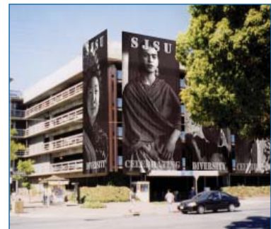
Before: the building as a parking garage
